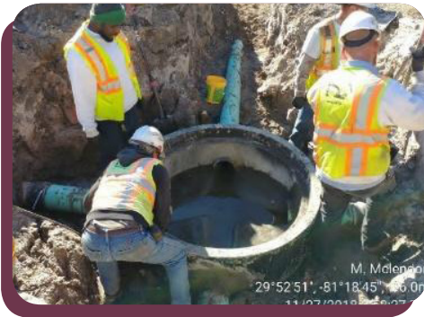
Workers install a manhole on Duero Street
