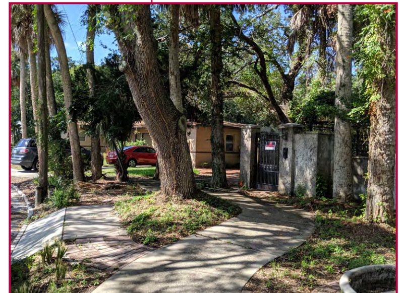
Sidewalk is in good condition. Existing trees beginning to lift sidewalk.
