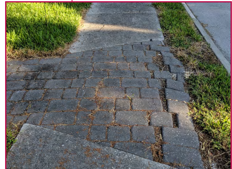
Damaged pavers within a good section of sidewalk.
