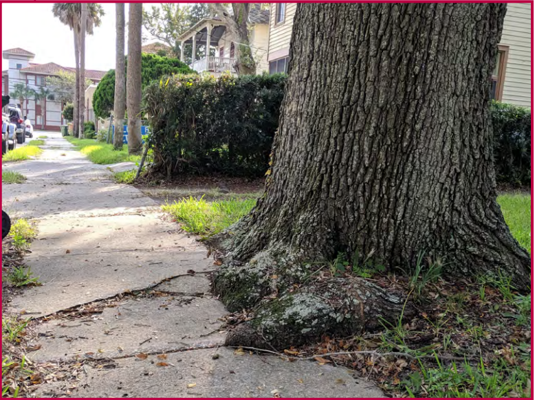
Large existing oak tree lifting/cracking sidewalk.
