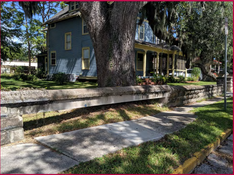
Previous sidewalk repair beginning to buckle/crack.
