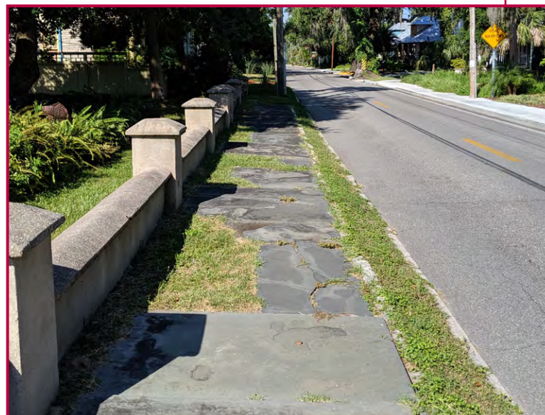
Existing slate sidewalk has broken/missing sections. Non-ADA accessible.
