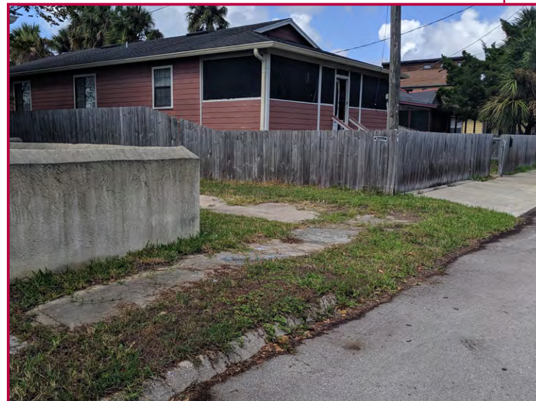
Broken/missing sections within a continuous section of good sidewalk.
