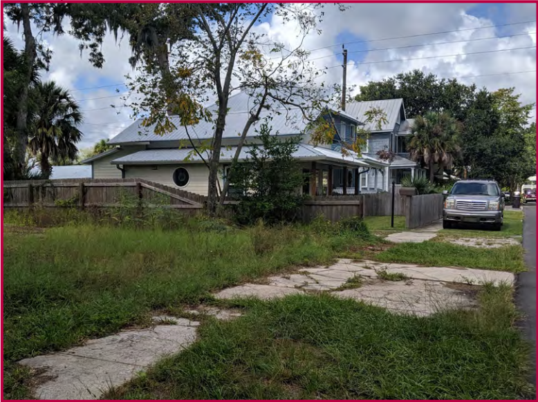
Existing tree lifting sidewalk with significant damage.
